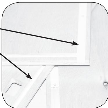
**IMPORTANT:** If you are going to use the CLEAR DOOR FLAPS, NOW would be a good time to install them as it is much easier to get a proper alignment. Simply remove the tape and stick the door flap above the door. After initial installation, they can be removed.
